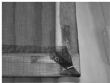
Figure 4. Attachment of screen to frame.
