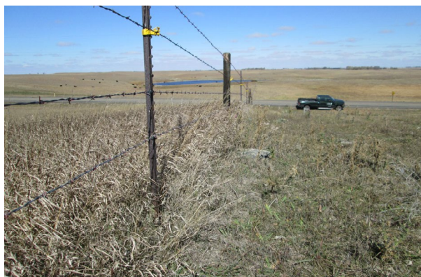
Figure 3: Modification of a four-strand barbed wire perimeter fence with an electrified 'hot' wire for additional negative reinforcement (left). Three to four-strand electrified high-tensile wire perimeter fences are becoming more common as materials and installation methods continue to be refined (right). Photo by Pete Bauman.
