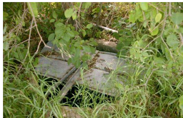
Figure 10: Isolated or abandoned pasture wells or old windmill pits can be refurbished for use under certain conditions, either with solar powered or 110V pump systems. Solar systems on wells where significant lift (>15 ft.) is necessary may require higher capacity solar panels and casing pumps to generate enough electricity to deliver adequate water volume for livestock ( photos by Pete Bauman ).
