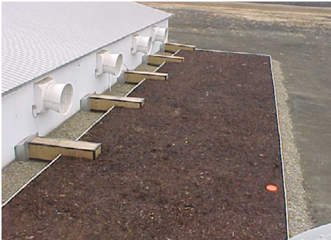
Figure 1. Odor control is critical for reducing the frequency of annoying odor events. Shown in this picture is a horizontal biofilter that treats exhaust air from pit fans.
