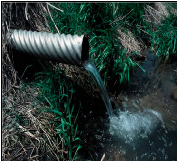
Figure 20.1. Water flowing from the outlet of a subsurface drain. (Photo by Lynn Betts, USDA Natural Resources Conservation Service)
