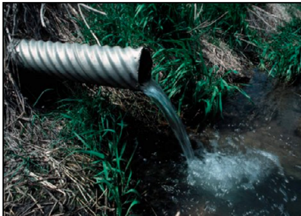
Figure 47.1. Water flowing from the outlet of a subsurface drain. (Photo courtesy of Lynn Betts, USDA Natural Resources Conservation Service)
