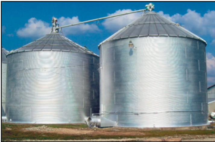
Figure 42.1. Grain bins need to be inspected regularly for pests.
