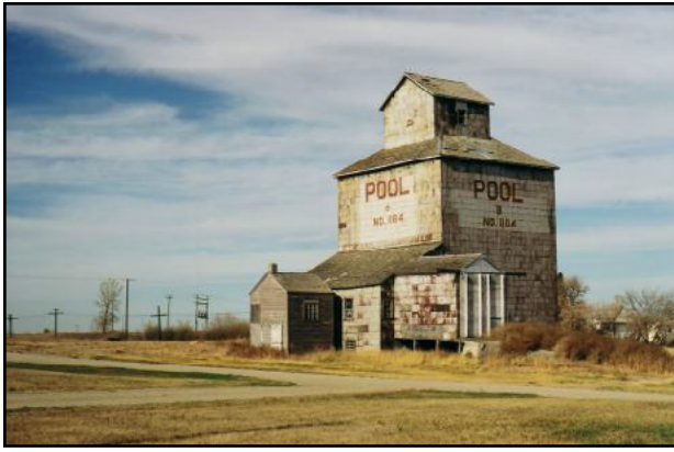
Figure 41.1. Grain elevator in Saskatchewan. (Source: http://esask.uregina.ca/entry/grain_elevators.html )
