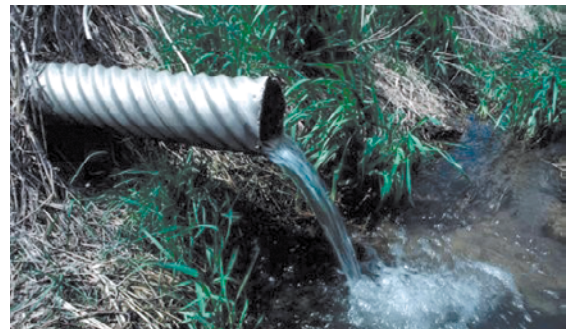
Figure 30.1 Water flowing from the outlet of a subsurface drain. (Photo courtesy of Lynn Betts, USDA Natural Resources Conservation Service)
